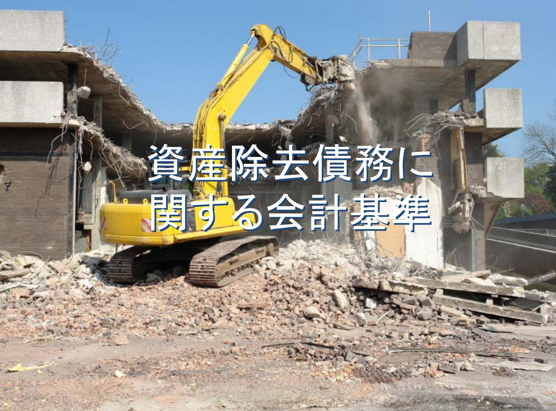
A yellow tracked excavator is shown in the process of demolishing a multi-story concrete building. The excavator's arm is extended, and it is actively breaking apart the structure, with dust and debris visible. The ground is covered in a large pile of rubble, including bricks, concrete blocks, and twisted metal. The sky is clear and blue. The text '資産除去債務に関する会計基準' is overlaid in the center of the image.
